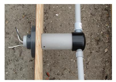
Orientation for installations where concrete gets a surface finish that is between 1/4" and 1" thick.
