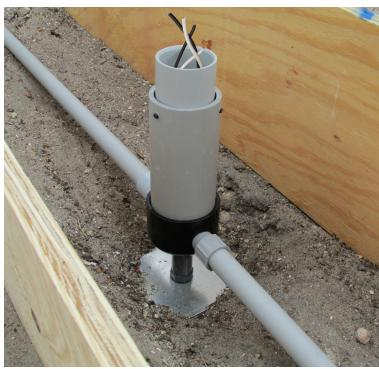
Orientation for vertical installations. Shown with optional junction box cover and pipe nipple (by others) used as a base and vertical extension. CFK may also rest directly on ground and PVC Pipe may be trimmed for even greater clearance for shallower pours.
