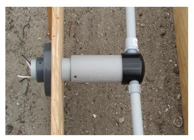
Orientation for installations with no surface finish material on the concrete or material that is less than 1/4" thick.
