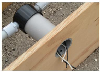
Orientation for installations where concrete gets a surface finish that is between 1" and 2-1/2" thick.
